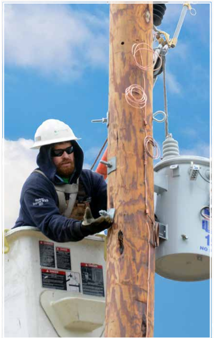
First-Class Line Technician Russ Drury works to install a new pole.
